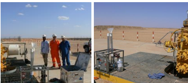
Fig. 1 – On site In Salah: RESMAN's current Norway OPS manager injected CCS tracers to monitor CO 2 movement from CCS injectors.
